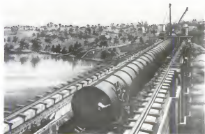
figure 53, right: Arthur Brown, High Bridge During Construction of the Large Main, Viewed from the West Gate House, looking East , 1861, three-color lithograph from Valentine's Manual Courtesy private collection. Photo: B. Sigler
